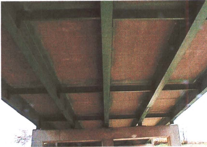
BOTTOM OF DECK
