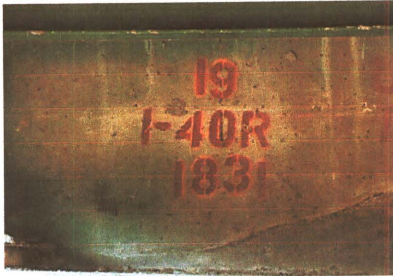
BRIDGE NO. AT ABUTMENT # 1
